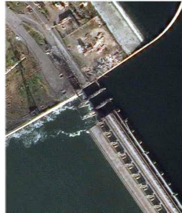
Figure 7. Satellite image of the damaged Kakhovka dam showing the damage to the roadway and dam on 11 November 2022 (Source: https://twitter.com/Maxar/status/1591158455808954368/photo/2 ).
