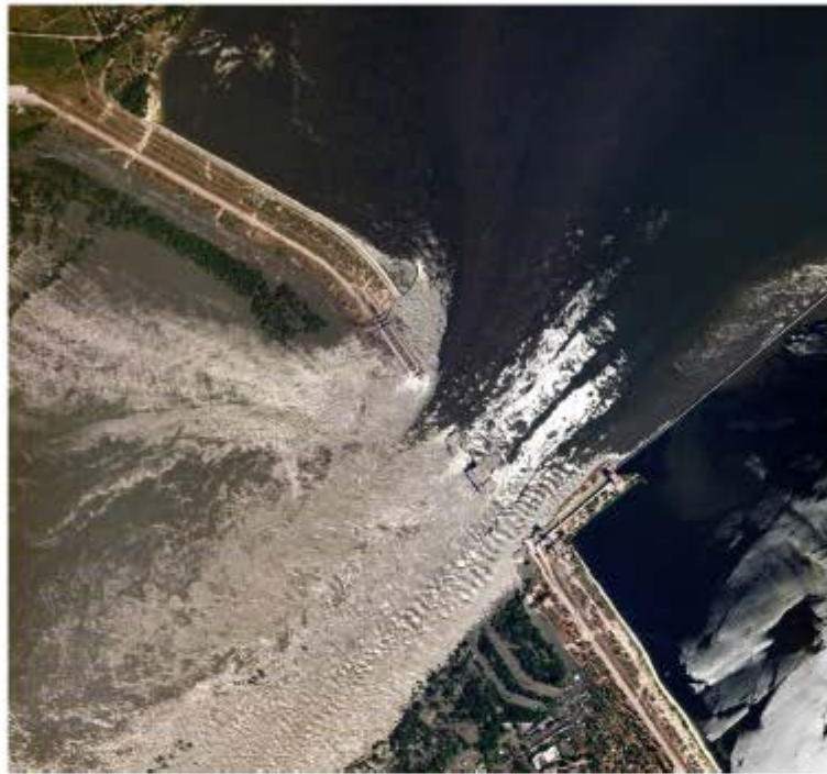
Figure 8. The destroyed Kakhowka facility on 6 June 2023 a few hours after the explosion (Source: https://twitter.com/GianlucaMezzo/status/1666097052269559816 ).
